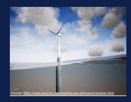
Concrete is used for floating offshore wind floaters and is expected to be important also in future installations. Requirements in current standards are based on experience from O&G and bottom-fixed structures.
